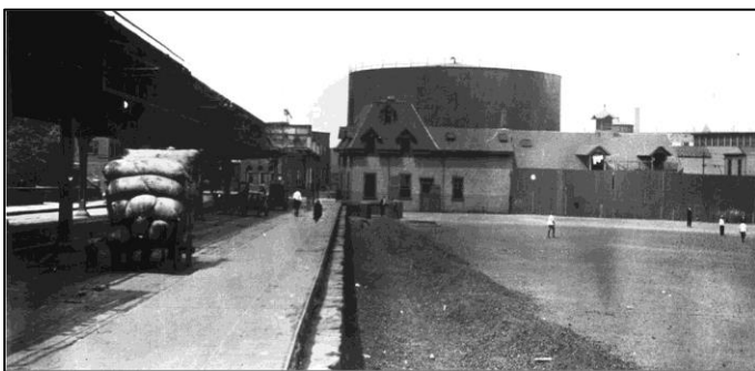
The molasses tank looms over Boston's Commercial Street
